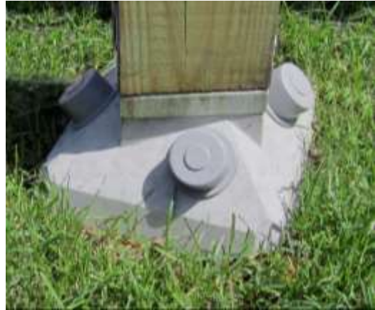
Figure 7. Completed Installation with Inspection Caps
