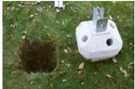
Figure 3. Tapered Hole for Concrete Head
