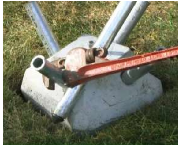
Figure 6. Jacking Method for Pin Removal
