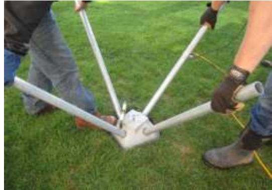
Figure 4. Setting Pins and Leveling Pier
